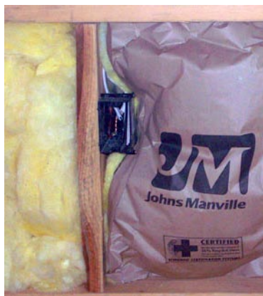
Figure 1.1. (left) Cut fiberglass batt insulation to fit around electrical boxes and wiring or pipes that run through the walls. Compressions like these ruin the batt's thermal alignment with walls and lessen its effectiveness.
